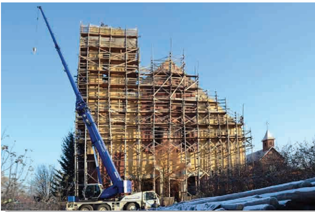
Erection of the cross on the church in Dęblin, Poland
