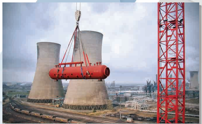
Waste incineration plant in Cleveland, UK
