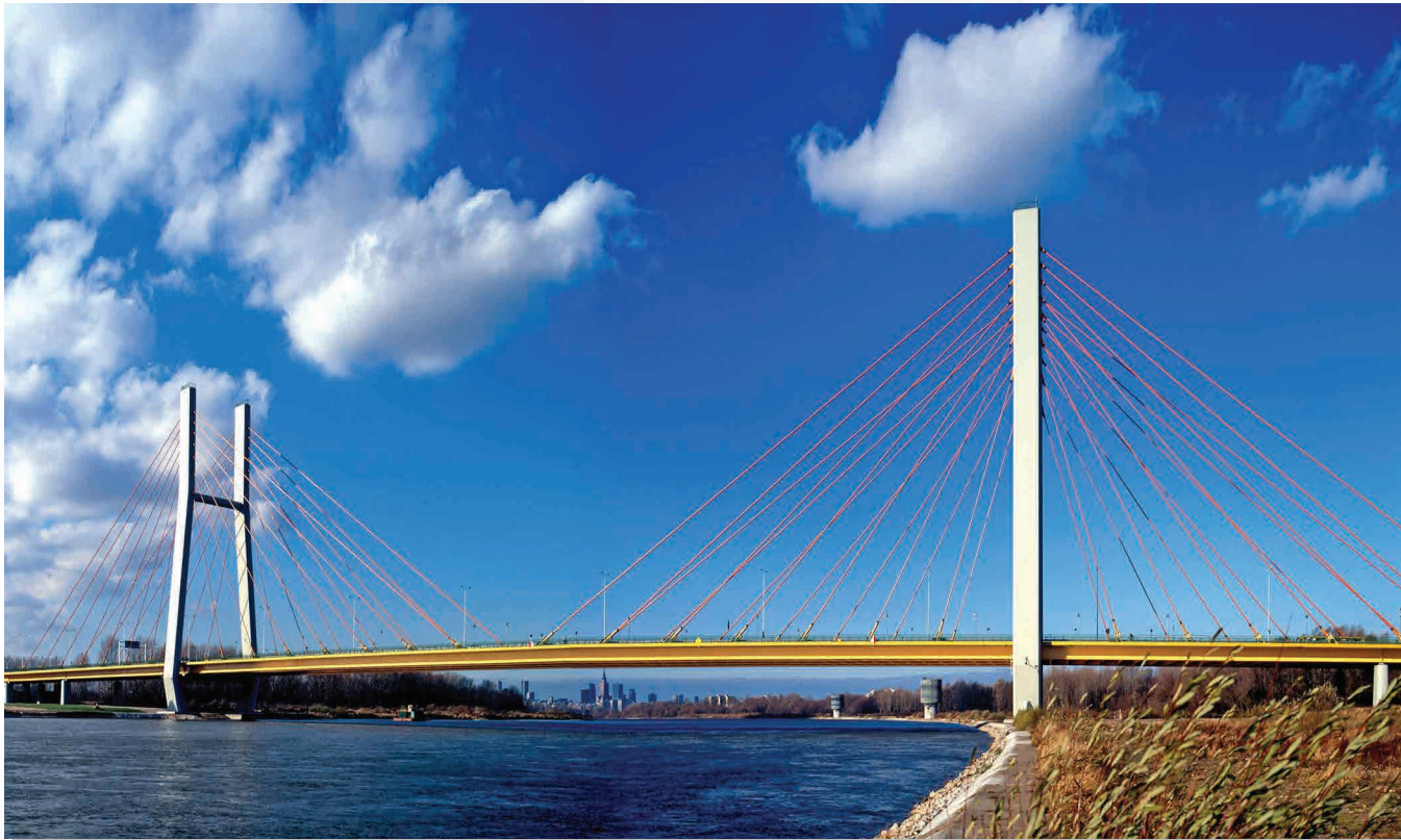
The Siekierkowski Bridge over the Vistula River in Warsaw, Poland
