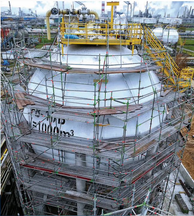
Spherical tanks for PKN Orlen in Plock, Poland
