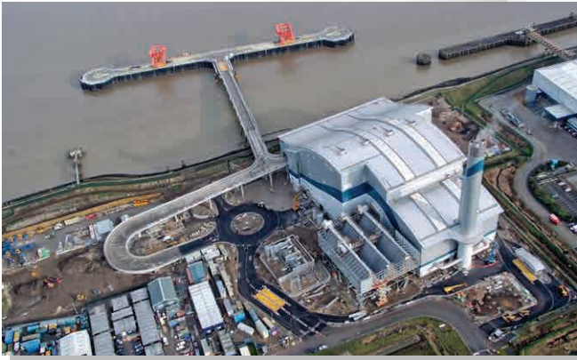
Riverside waste incineration plant in the south-eastern part of London, UK
