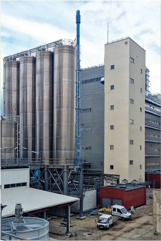
POLYAMIDES II Plant in Tarnów, Poland
