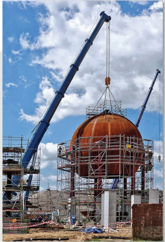
Spherical tanks for PKN Orlen in Plock, Poland
