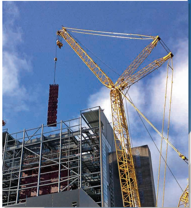
Erection of CFB boiler at CHP plant in Jyväskylä, Finland
