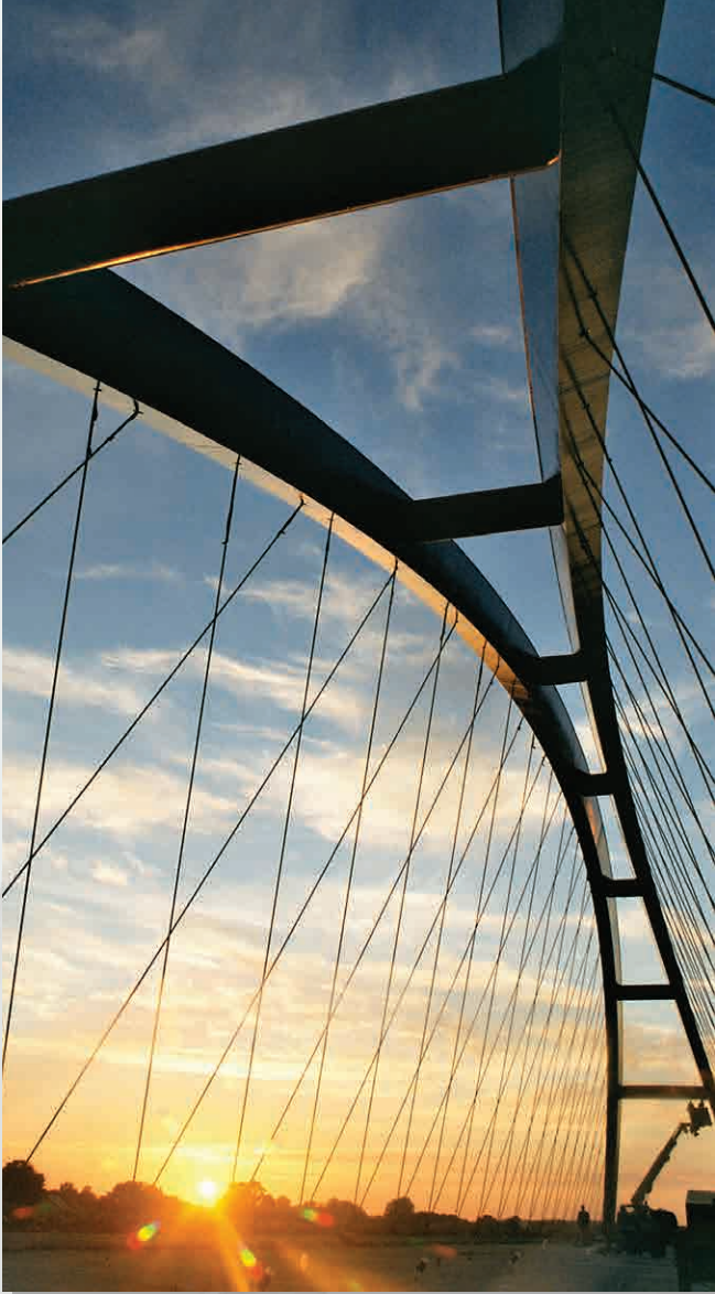
Bridge over Dziwna River in Wolin, Poland
