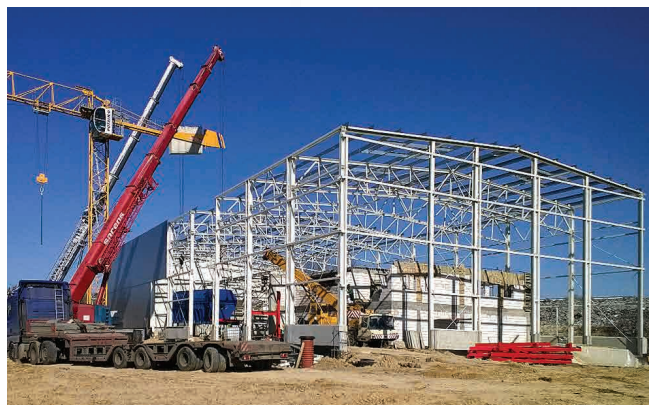
Regional Waste Management Plant in Dębowiec, Poland
