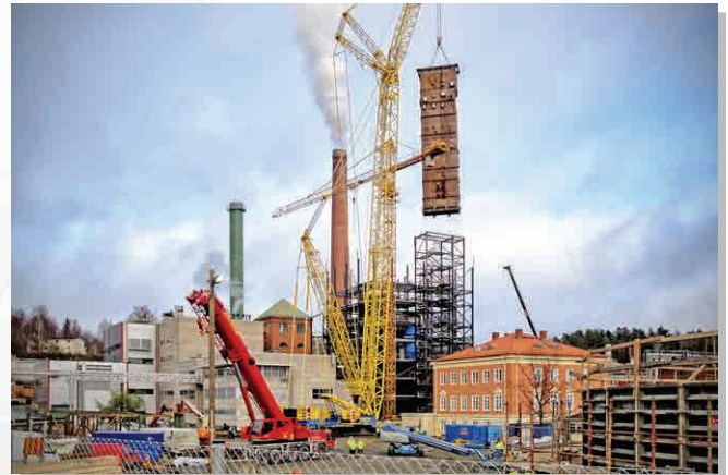
Erection of BFB boiler in Havo CHP plant, Finland
