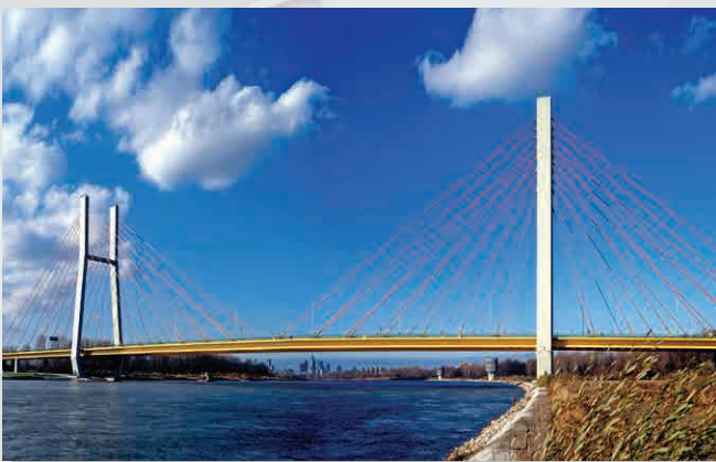
The Siekierkowski Bridge over the Vistula River in Warsaw, Poland
