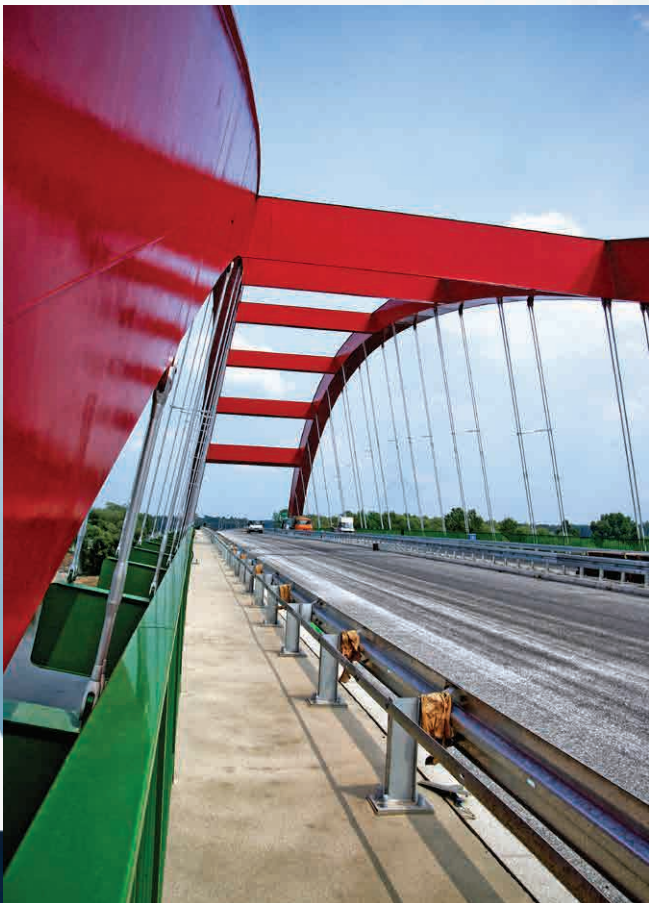
The John Paul II Bridge over the Vistula River in Puławy, Poland
