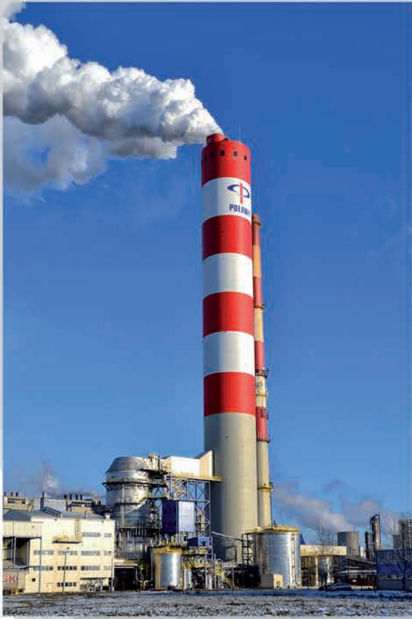
Construction of flue gas desulphurisation plant at Zakłady Azotowe "Puławy" S.A., Poland
