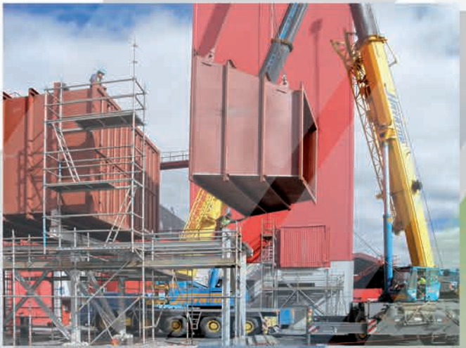
Supply, steel structure erection and thermal insulation of gas cleaning plant for iron-ore pelletisation furnace at LKAB Svappavaara mine, Sweden
