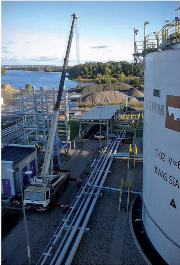
Upgrade of sulphuric acid terminal in Szczecin, Poland
