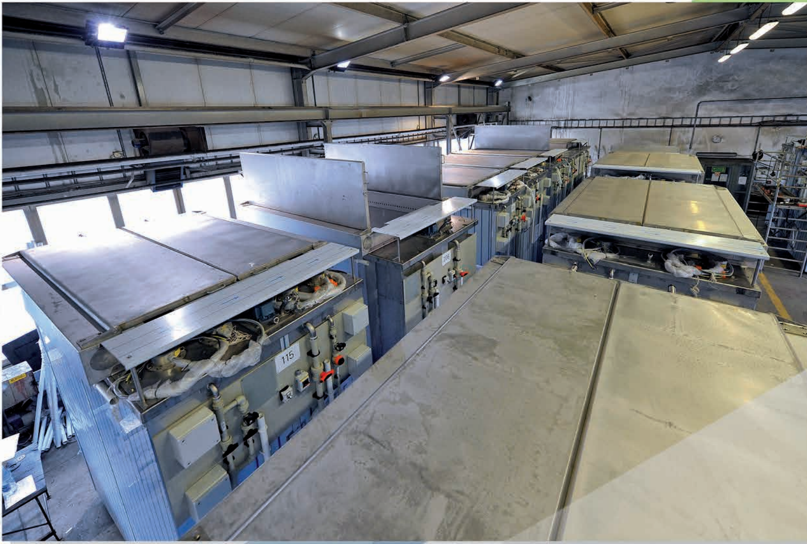
Manufacture of galvanising tanks for General Electric in the United Arab Emirates
