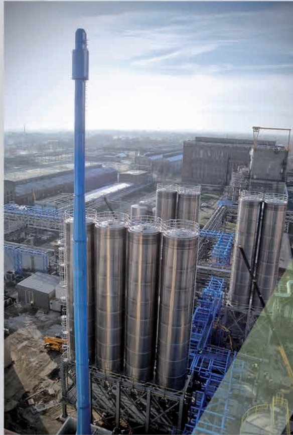
Construction and installation of pipelines (247 tonnes) and installation of apparatuses (263 pcs) at Polyamides II Plant of Grupa Azoty S.A. in Tarnów, Poland
