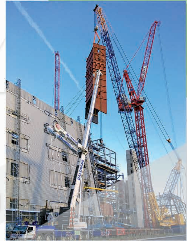
Erection of pressure parts of two boilers (62.6 MW th ) at Severnside waste incineration plant (capacity 388 000 t/year) in Bristol, UK
