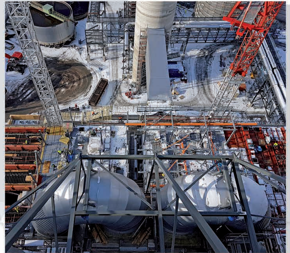
Installation of five ESPs for new bio-product plant owned by Metsä Fibre Oy in Äänekoski, Finland
