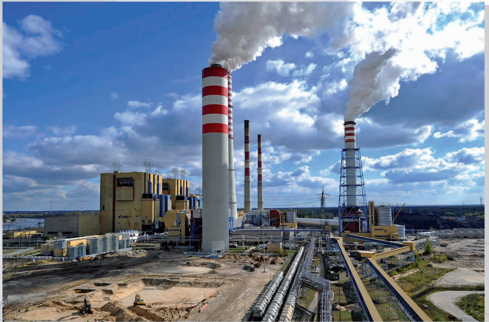
Upgrade of the fly and bottom ash hydraulic transport trestle bridge and return water pipelines from storage yard at Kozenice Power Plant, Poland
