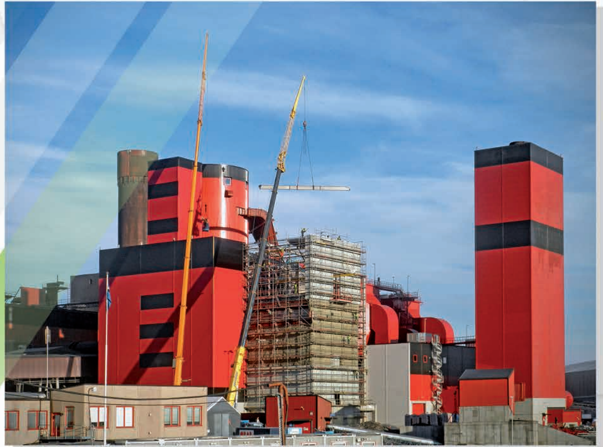
Supply, steel structure erection and thermal insulation of gas cleaning plant for iron-ore pelletisation furnace at LKAB Svappavaara mine, Sweden
